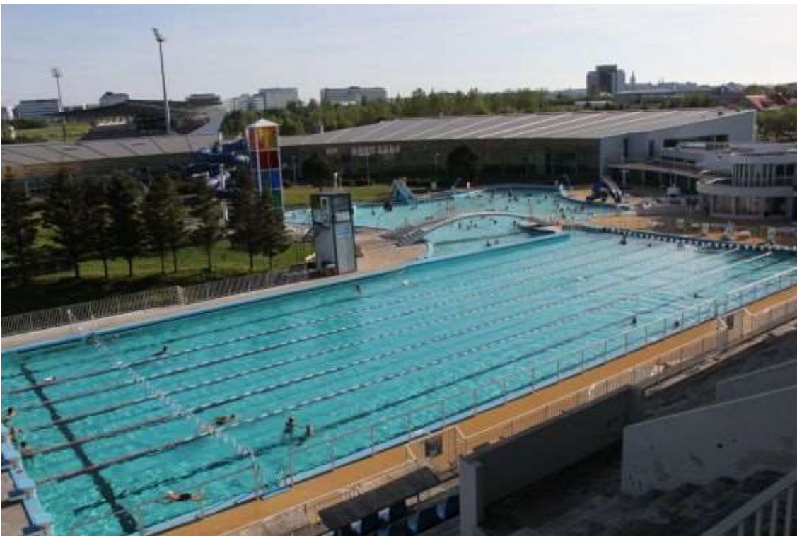
The Laugardal geothermal outdoor swimming pool – 50m, 8 lanes
